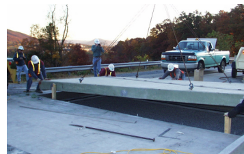
Use of fiber reinforced polymer deck panels for rapid repair of bridge structures.
